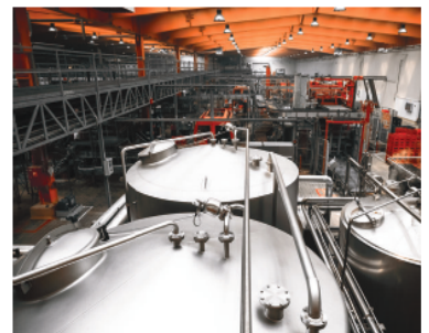
Millions of dollars are lost every year in the food and beverage industry from production line damage and lost productivity when hoses and wires are damaged by rodents.
